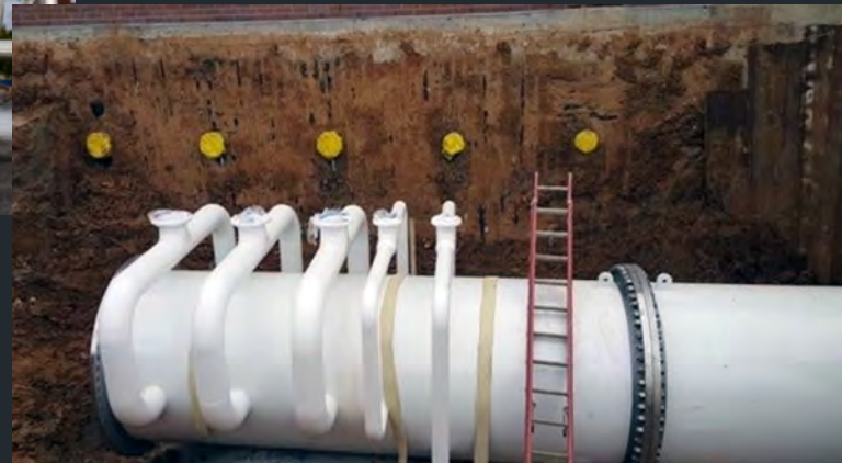
Pipeline Flash Reactor - buried
