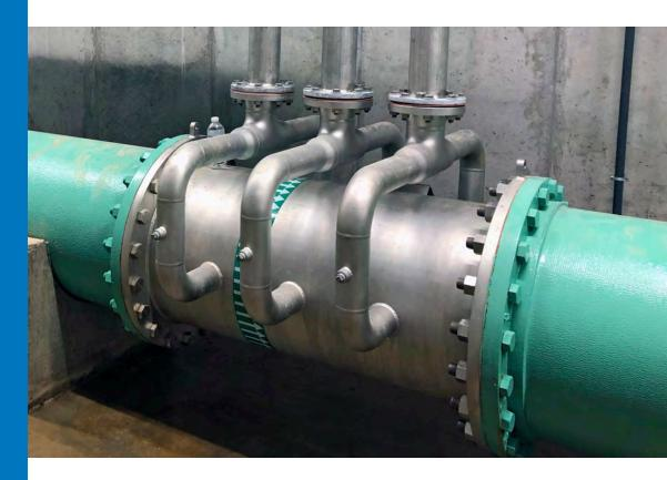
**THE RESULT:** After (3) years of operation, plant personnel confirmed that only minimal, routine maintenance had so far been required. Along with the other upgrades completed as part of the plant improvement project, the installation of the new oxygen injection system has enabled the plant to reduce THM levels by 40% - 50%, improve the DAF's efficiency, and expand treatment capacity to 8 MGD, all without adding to the daily responsibilities of plant personnel.
