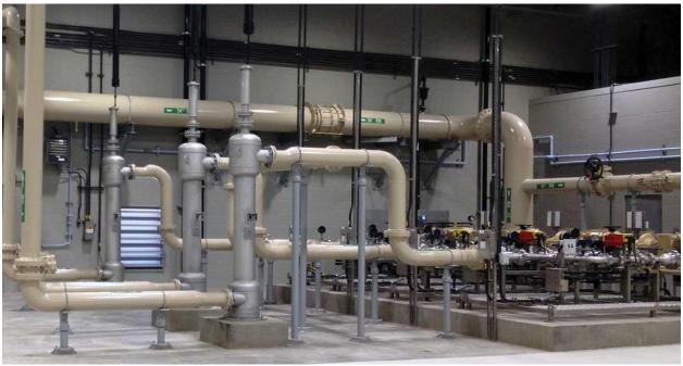
The San Angelo, Texas facility selected the Mazzei GDT system, which aerates a sidestream using venturi injectors and a Pipeline Flash Reactor (PFR) to blend the treated sidestream effectively as it is reintroduced into the main flow. Photo courtesy of Mazzei Injector Company
