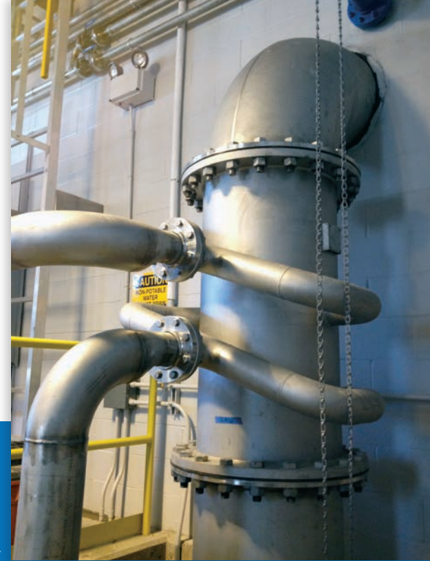
FIGURE 1: Pipeline Flash Reactor
