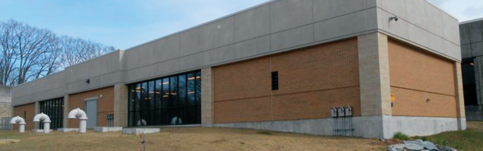
Vernon C Russell WTP Phase II Facility
