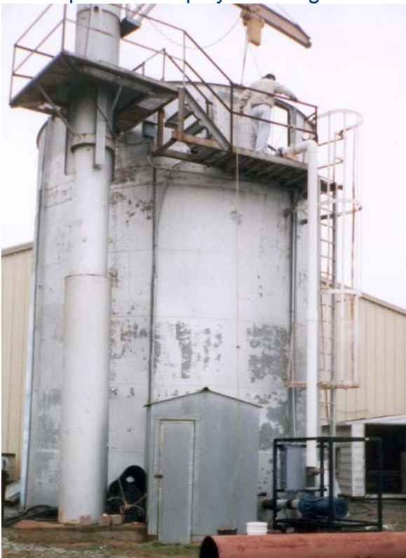
Test Tank 21' Diameter x 30' Deep & Circulation Pump
