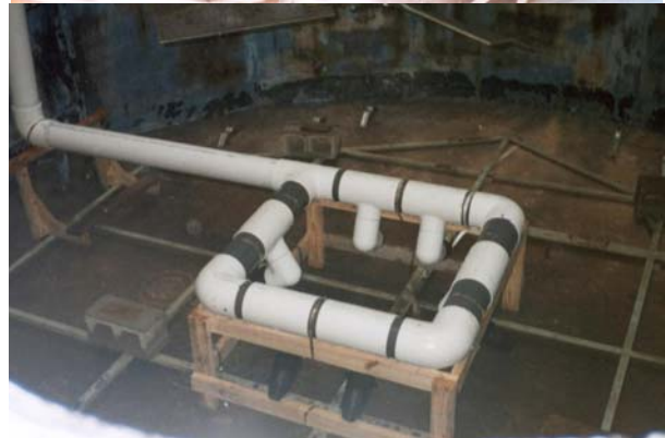
Mazzei N45 Nozzles & Manifold
