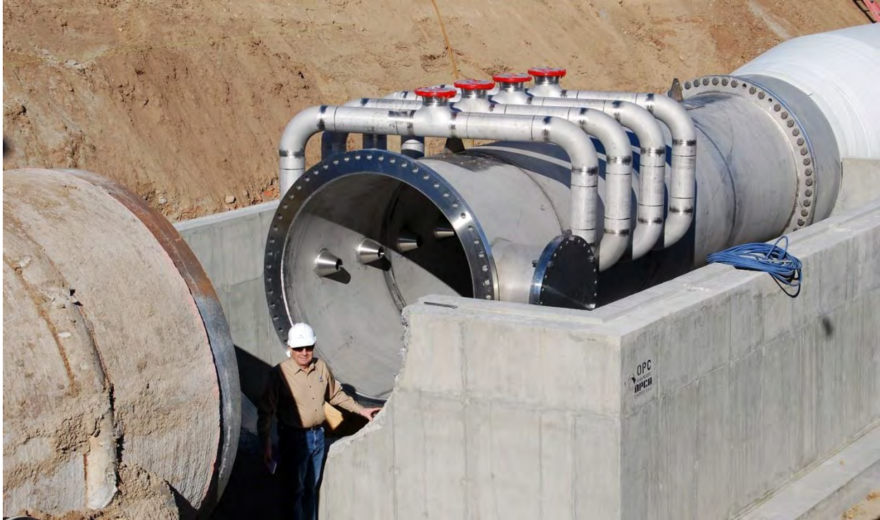
IMAGE 3: Angelo Mazzei pictured with a Pipeline Flash Reactor (PFR) at a water treatment plant in Castaic, California (10 – 140 MGD capacity). In just a few feet of pipe, specially engineered and oriented mixing nozzles blend ozonated sidestream into the main flow.
