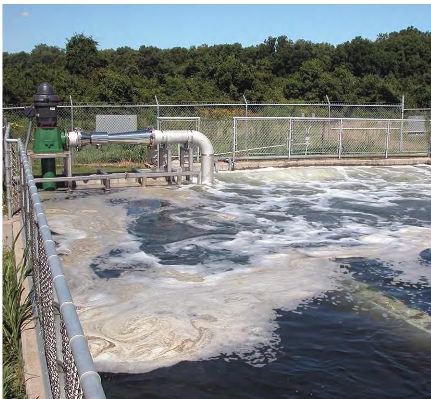
IMAGE 1: A single pump and Venturi injector efficiently aerate a basin. Basin aeration is especially effective for treating effluent with high levels of solids. (Images courtesy of Mazzei Injector Company)
