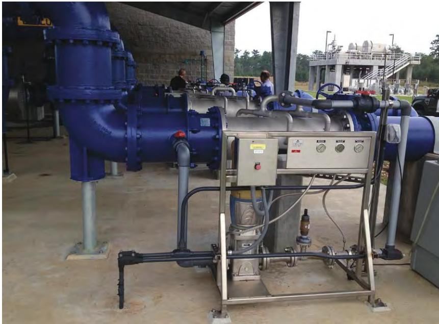
IMAGE 2: In just a matter of a couple of feet, the silver-colored pipeline flash reactors at this water treatment facility shear and mix a sidestream flow that has been aerated by passing through a venturi injector (bottom, on skid).
