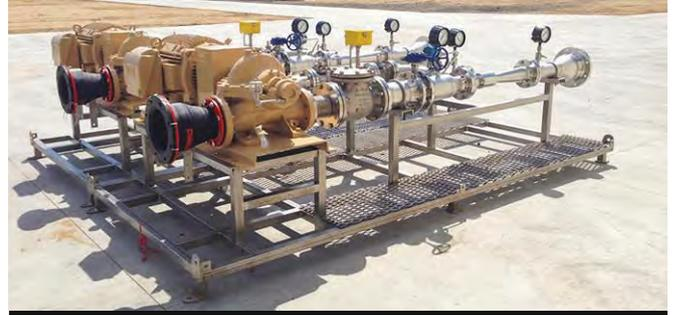
Image 1. Platform-mounted injector systems aerate water in the Hickory Aquifer Groundwater Treatment Facility in San Angelo, Texas, to remove dissolved iron. Shown are two of the four sidestream aeration systems. (Images courtesy of Mazzei)
