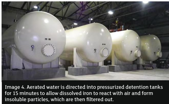
Image 4. Aerated water is directed into pressurized detention tanks for 15 minutes to allow dissolved iron to react with air and form insoluble particles, which are then filtered out.
