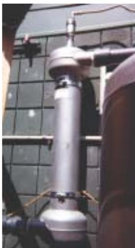
Photo 1. Degas separator used on a water stream prior to the water entering a zoo's hippo exhibit
