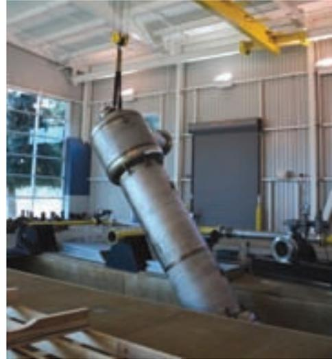
**Figure 3.** Seating degas separator into sump.
