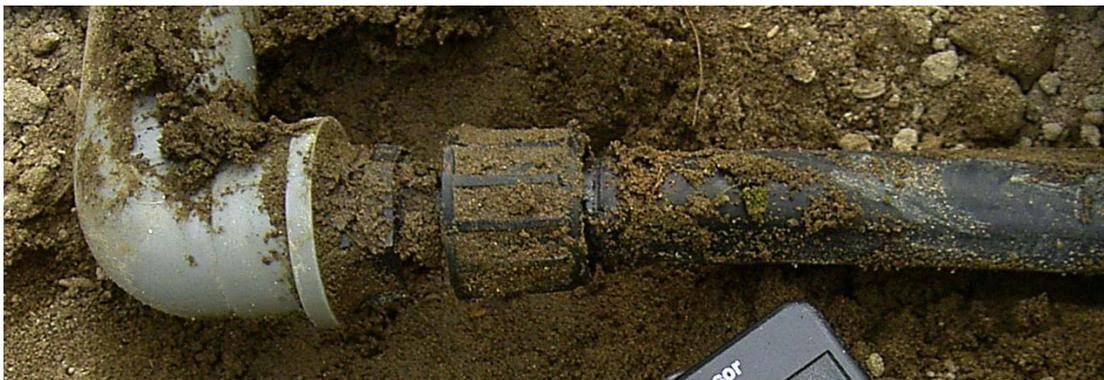
Irrigation tubes and regular water equipment joints were connected with a special tubing adaptor. This system will be applicable with other standardized parts, provided that the diameter and thickness are same.
