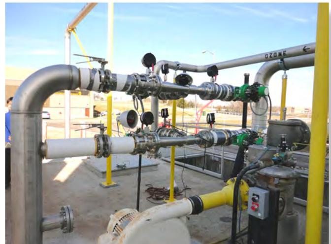
*To get a better understanding about how a [Mazzei Sidestream Venturi Injector-Basin Nozzle Manifold](#) system works, take a look at this [animation](#).*
