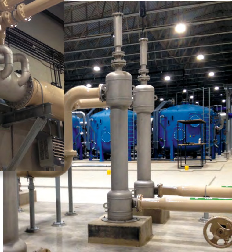
FIGURE 4. Degas Separators
