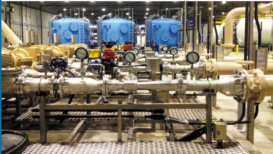
FIGURE 1. Venturi injector in GDT/PFR train
