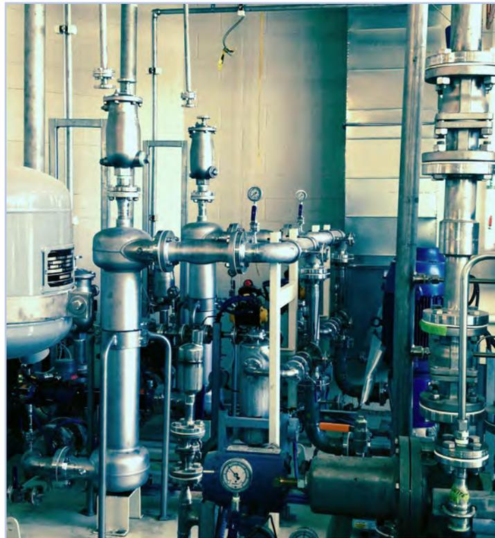
FIGURE 1: GDT Ozone Contacting Skids at Buckingham WTP
