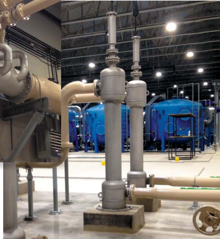
FIGURE 4. Degas Separators
