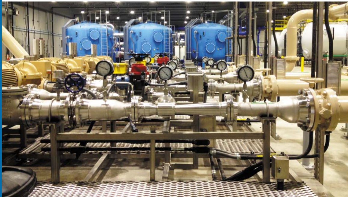
FIGURE 1. Venturi injector in GDT/PFR train
