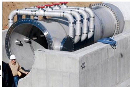
Mazzei's innovative Pipeline Flash Reactor — now fine-tuned with state-of-the-art computational fluid dynamics (CFD) modeling — packs powerful mixing and shearing action into an area only the length of 3 to 5 diameters of the mainstream pipeline.
