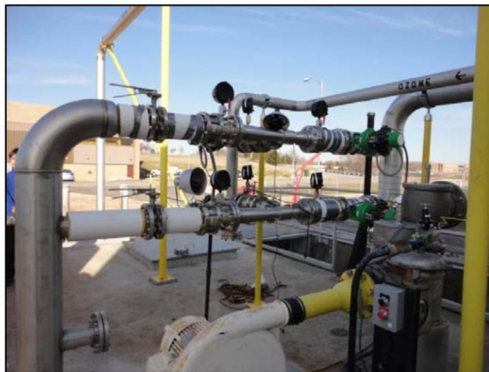
Figure 4. Contactor No. 3 ozone injectors
