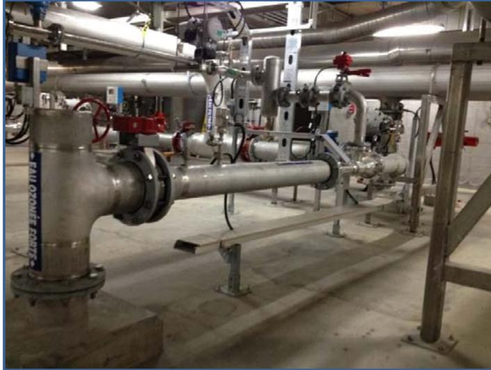
Figure 13. Des Baillets sidestream Mazzei injectors.
