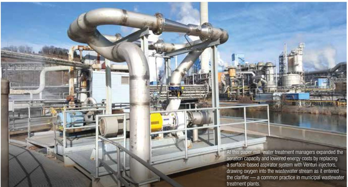
At this paper mill, water treatment managers expanded the aeration capacity and lowered energy costs by replacing a surface-based aspirator system with Venturi injectors, drawing oxygen into the wastewater stream as it entered the clarifier — a common practice in municipal wastewater treatment plants.
