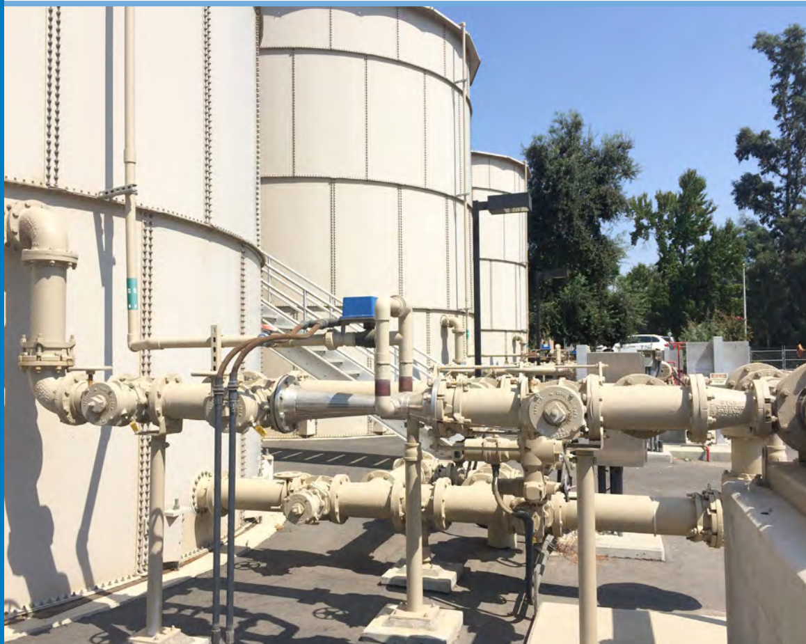
Reedley Wastewater Treatment Plant
