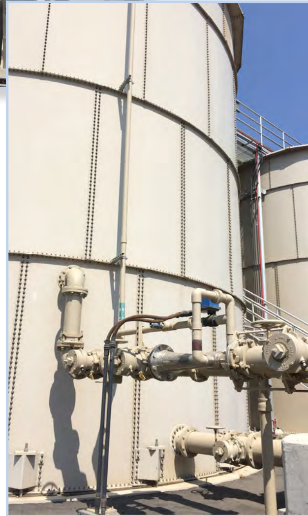
Reedley Wastewater Treatment Plant
