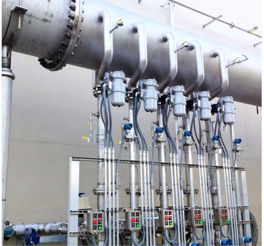
Retrofit installation of a gas diffusion contact basin. Five vertical Mazzei® Venturi injectors discharge up into a Pipeline Flash Reactor™ to treat up to 45 MGD. The equipment replaces the 552 diffusion stones that were taken out of service.
